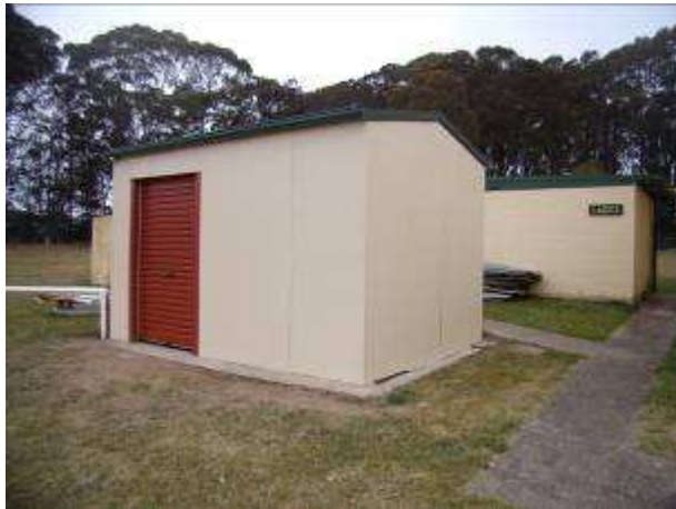
The new Storage Shed
